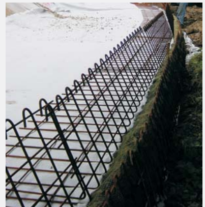
Placement of the formwork for the next layer
