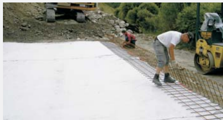
Placement of formwork elements
