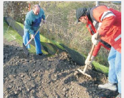
Installation and compaction of the topsoil along the slope surface by hand
