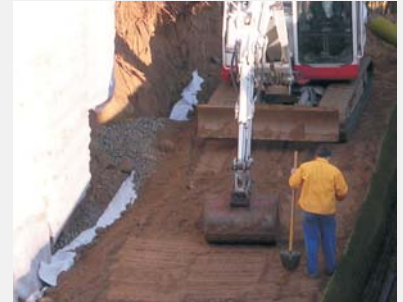
Drainage behind the reinforced earth structure
