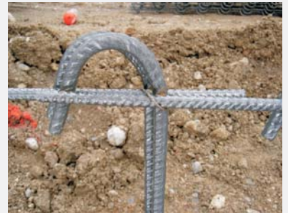
Connecting the rods at overlaps
