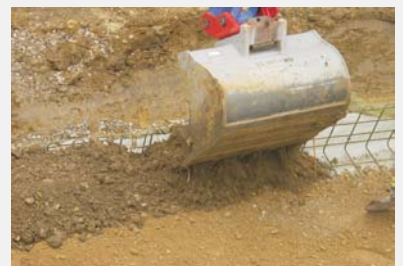
Fill of topsoil along the edge of the slope
