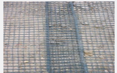
Placement and overlap of reinforcement geosynthetic
