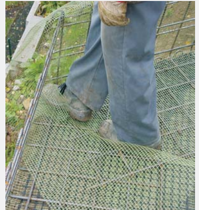
Careful placement of the erosion-protection grid
