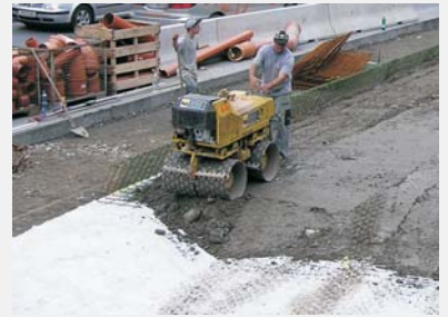
Compaction of the boundary strip
