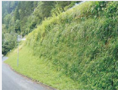
Vegetation applied by hydroseeding
