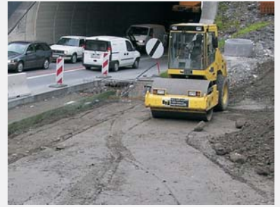
Compaction of the rear part of the slope
